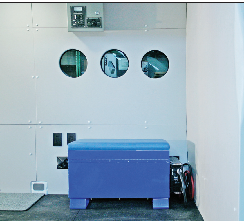
Porthole Windows and Battery Box
